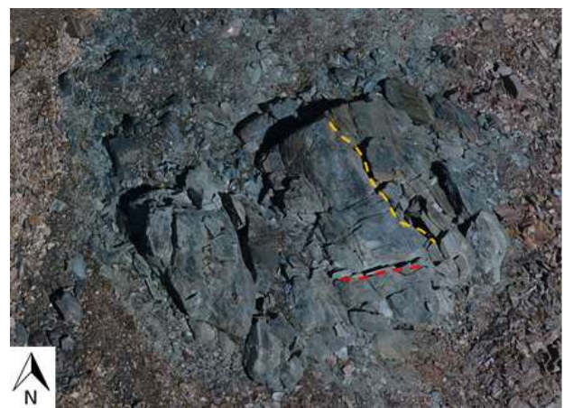
Figure 2: Outcrop of metabasite in which are visible the two fracture families: NW-SE (yellow hatch) and NE-SW (red hatch) (nadiral image by IMAGEO S.r.l) (coord. 412035.9, 5081194.5)
